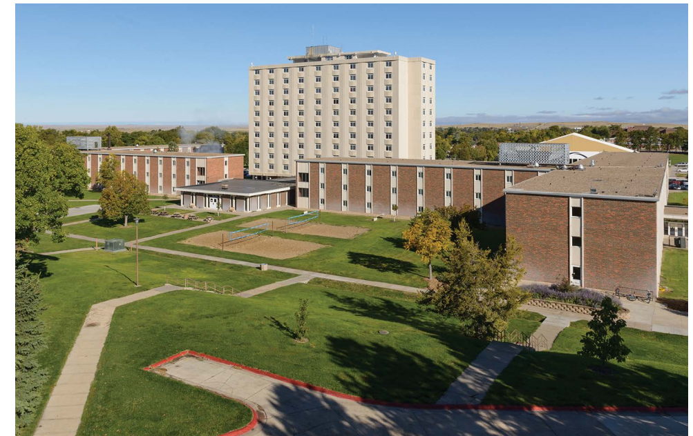
High Rise flanked by Kent Hall to the left and Andrews Hall to the right in this October 2017 view from the Math Science building roof. (Photo by Daniel Binkard)
