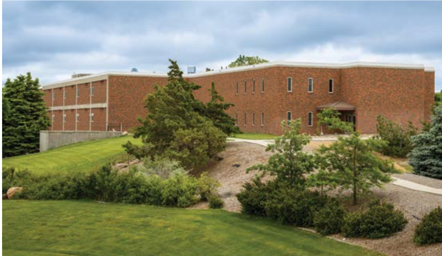
Construction is expected to begin in the summer of 2020 for Chadron State College's Math Science building's renovation and addition. (Photo by Daniel Binkard)
