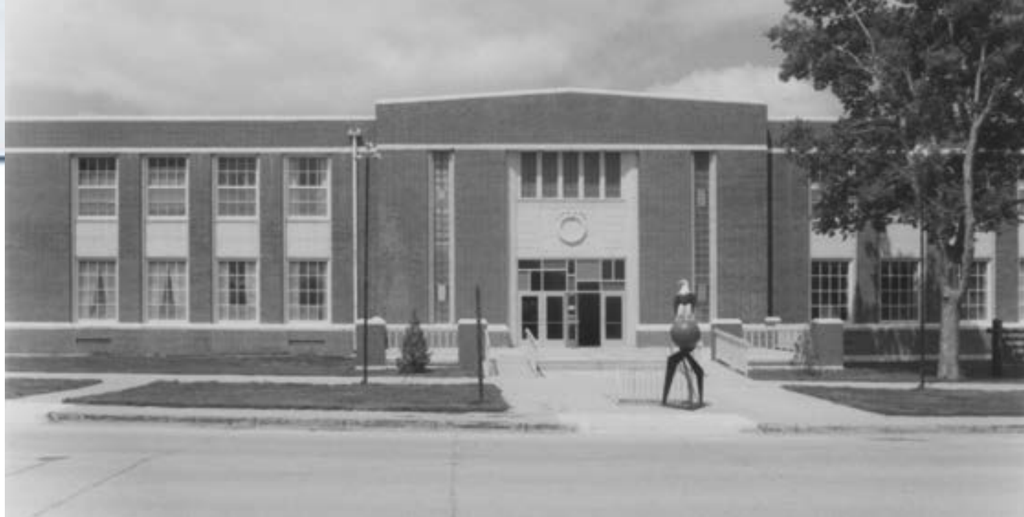
Memorial Hall has served many students and employees in a variety of capacities since it was built in the early 1950s. (Chadron State College Historical Photo)
